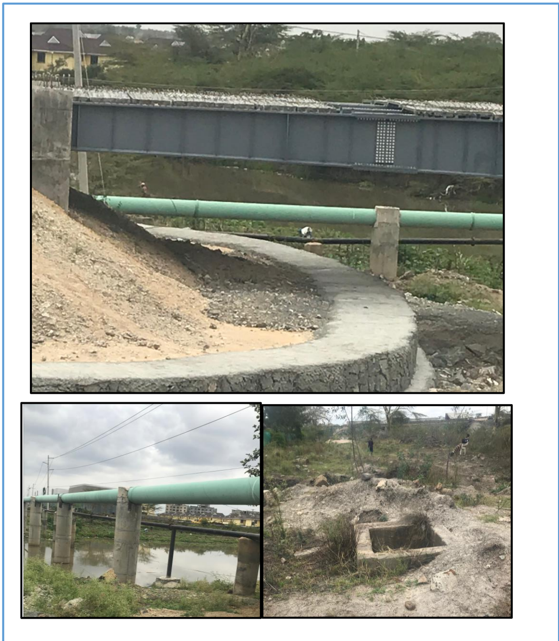
Plate 5: Infrastructure Facilities on Riparian Zones (source; Field 2019)
