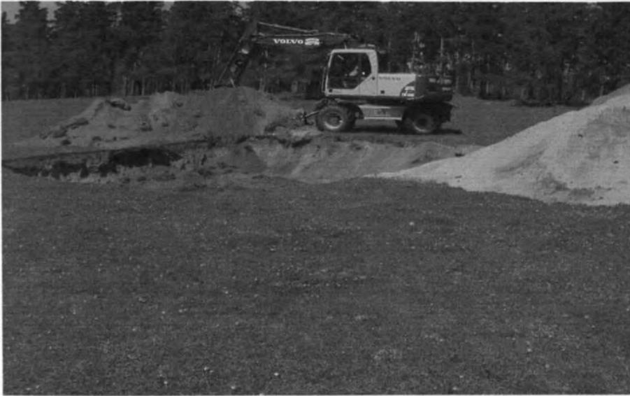
Plate 4: creation of 8 x 8 m plots and soil mixing
