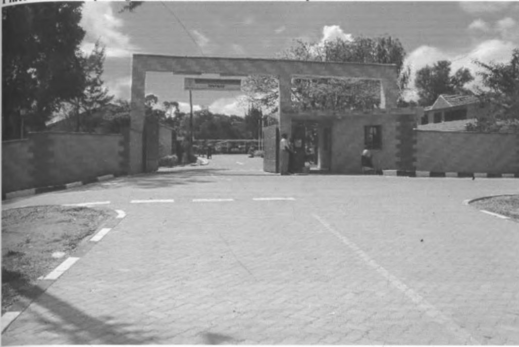
Plate 6.1: Roads paving outside within Mavoko municipal offices
