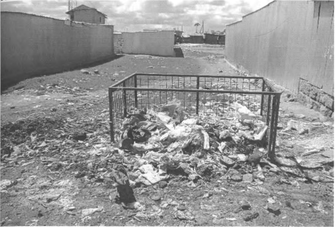
Plate 6.6: Poor maintenance of waste collection facilities
