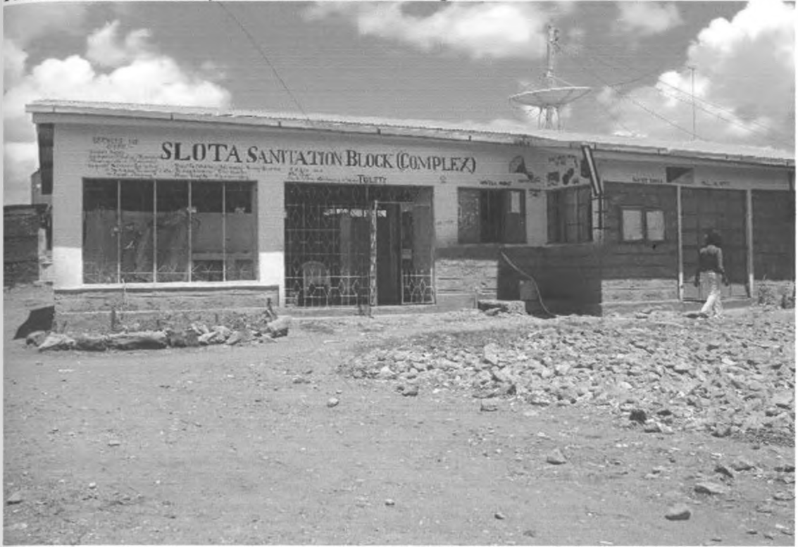
Plate 6.5: Slota community sanitation block and meeting hall
