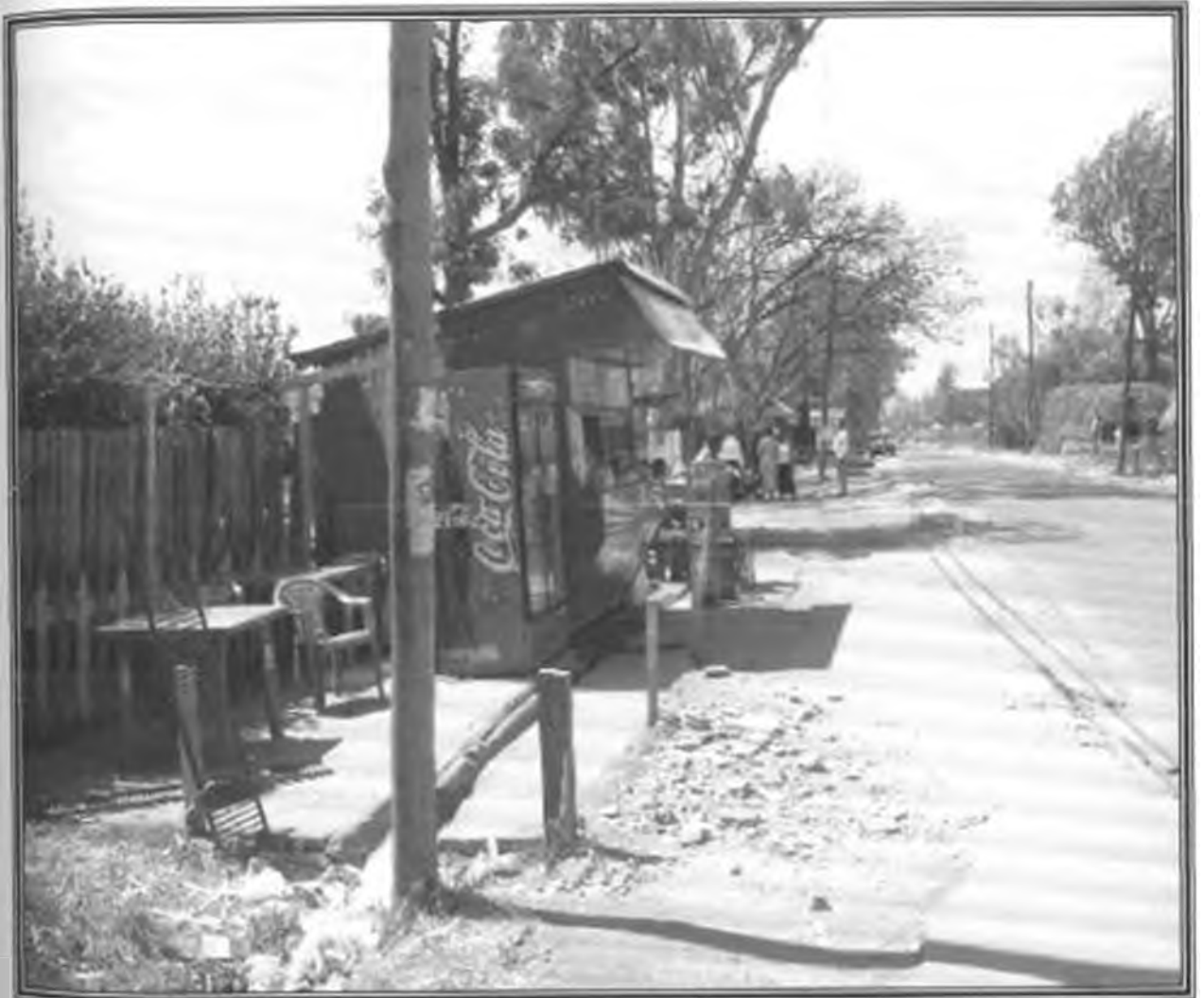
Plate 4.2: Poor development control - A Kiosk located on road reserve
