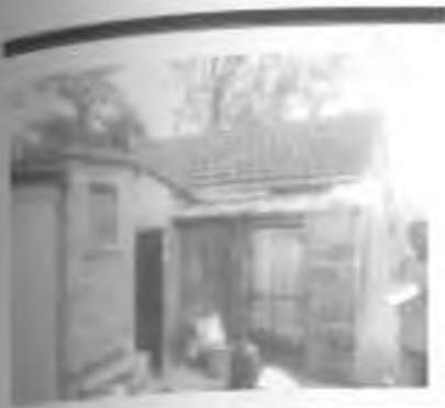
Figure 4-18: External view of L22 Source: survey, 2010
