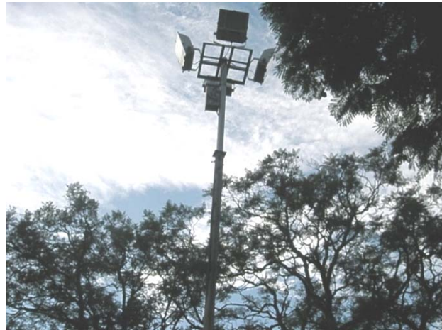
High level security lighting is good for this park
