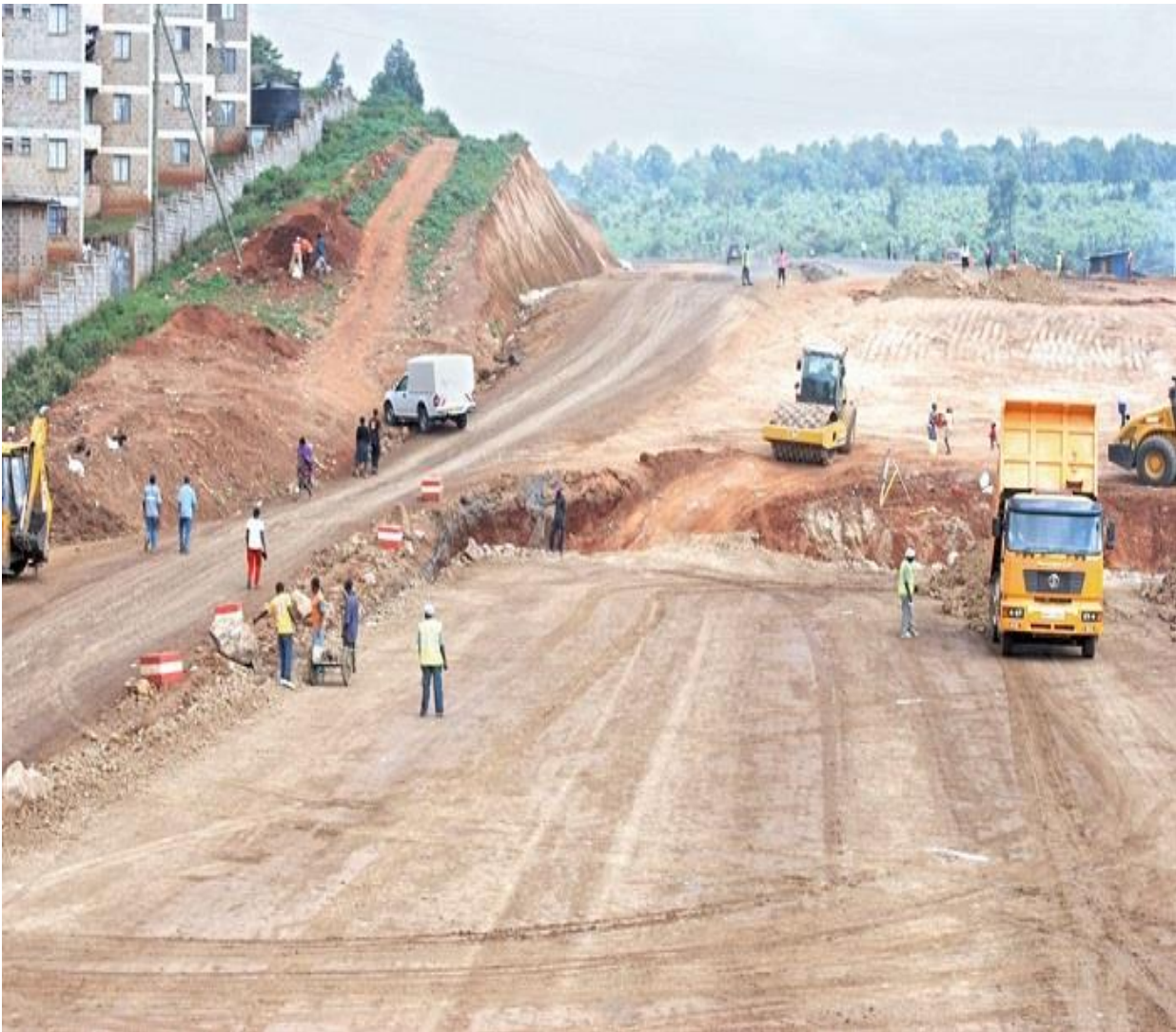
APPENDIX V Figure 4.4.5.2.2: Ongoing Infrastructure Project
