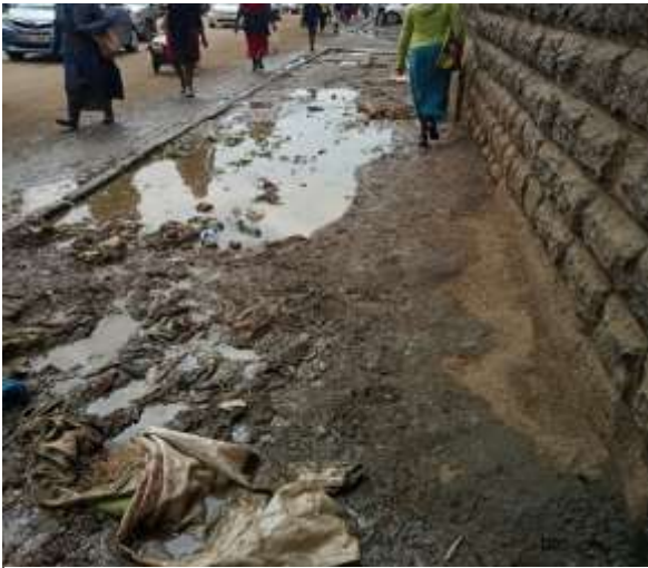
Plate 17: Poor state of pedestrian walk ways
