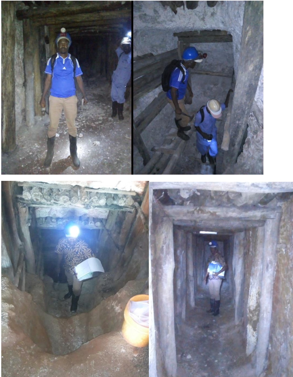
Figure 3. 3 Gallery (Adit) with Wooden Support
