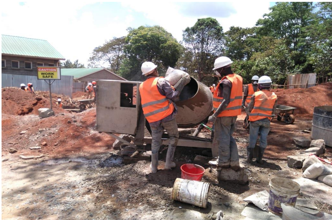
Plate 4.1: Concreting operation in progress at a site in Nairobi.
