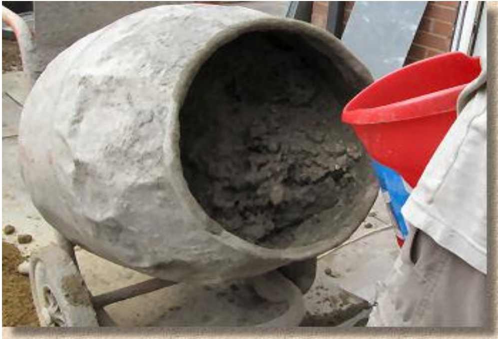
Plate 2.2: Basic concrete mixing equipment
