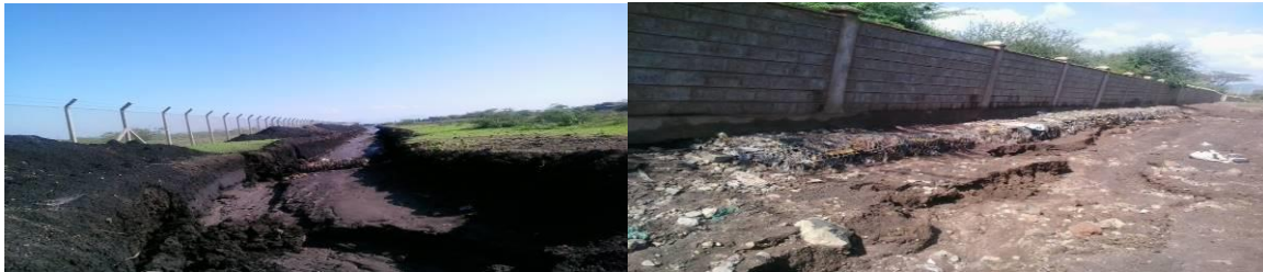
Opening up of flood channels along airport fence by Isiolo; d) Gabions built to reinforce the fence at Isiolo Girls Secondary school.
