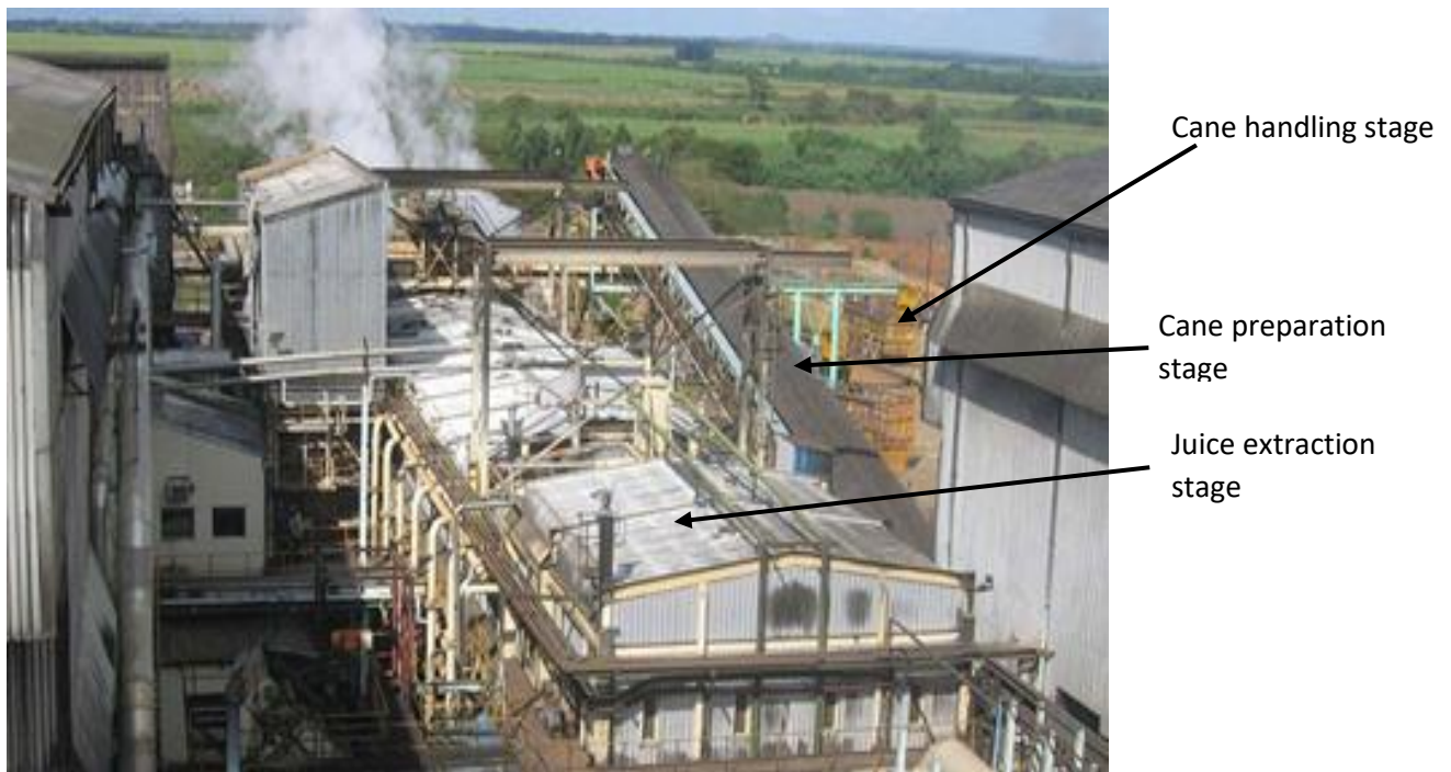
Figure 1-1: Pre-milling section at Mumias Sugar Company Ltd (MSCL, 2012)
