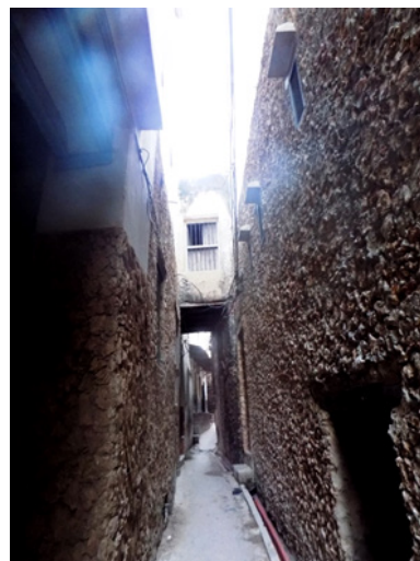
FIGURE 4 Image showing a wikio connecting two buildings in the enclave of Mkomani in Lamu Source: Author 2016
