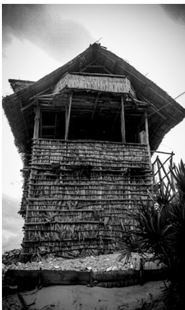
FIGURE 9 Image showing thatch and wattle structures in parts of Shela Source: Author 2016
