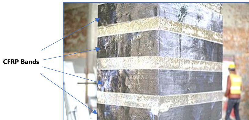
Figure 2.3: Partial CFRP confinement of a column.
