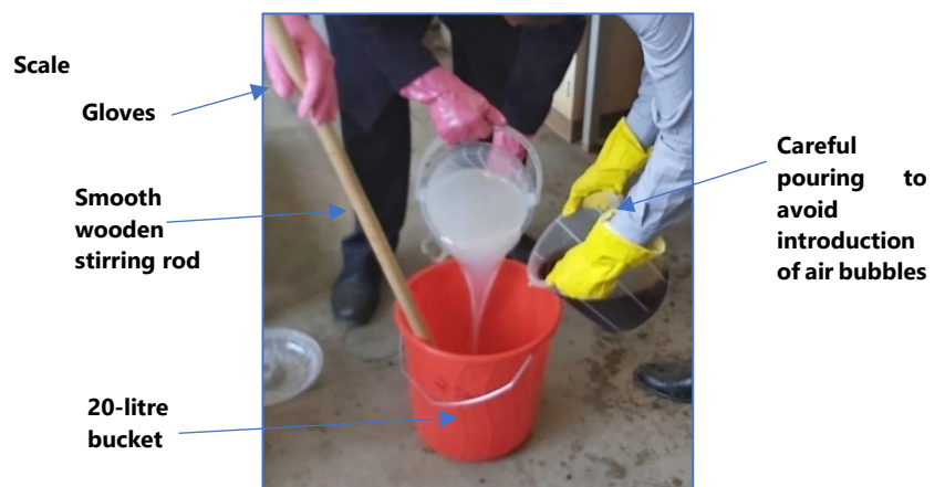
Figure 3.16: Mixing of the epoxy set with the ratio of 2:1.
