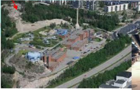
Viikinki Sewage Treatment Plant
