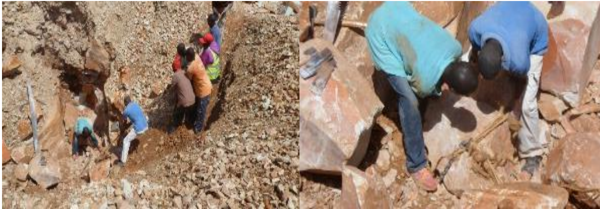
Plate 5.3: Extraction of Building Stones at Tabaka in Kisii
