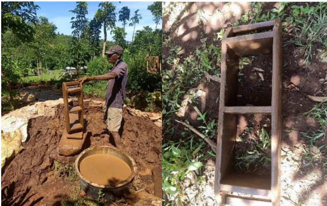
Plate 4.1: Material Preparation and Moulding of Bricks
