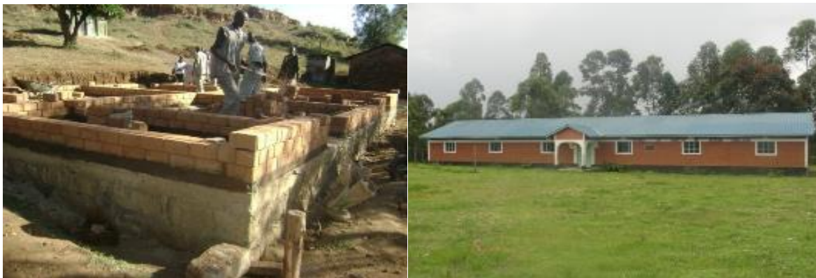
Plate 2.2 ISSB Construction Process and Completed Building with ISS Blocks.
