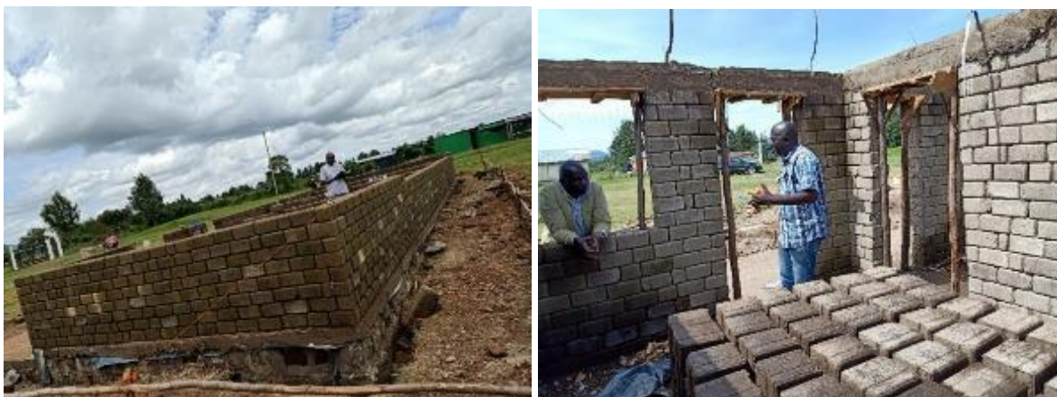
Plate 5.14: Mortarless Construction Using ISSB with Less Sequestered Energy
