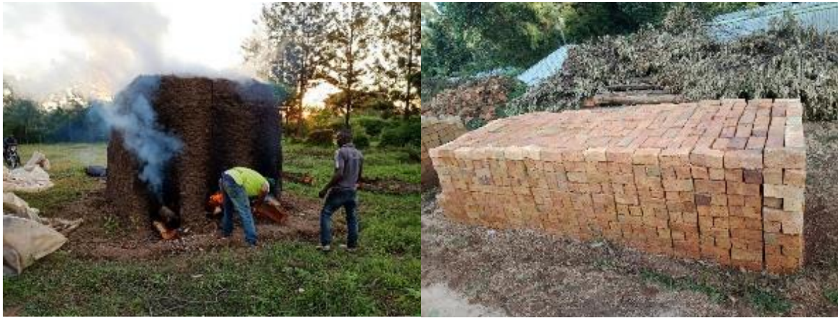
Plate 5.5: Firing of Bricks in readiness for Construction
