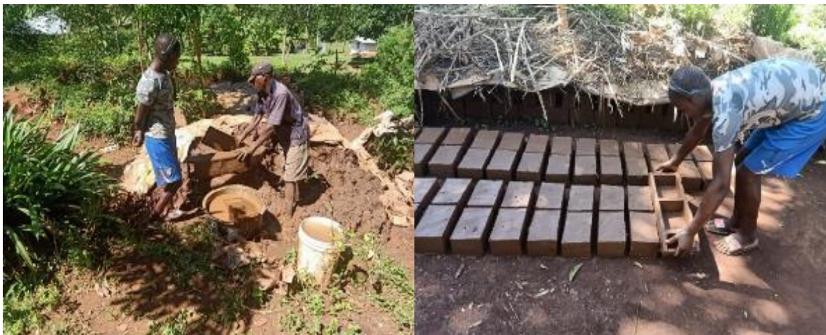
Plate 5.4: Moulding of Bricks during Manufacturing
