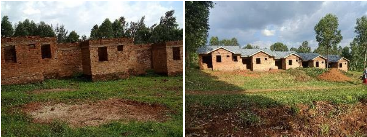
Plate 5.9: Town Estate Under Construction with Burnt Bricks in Rongo, Migori County
