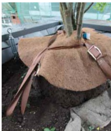
Figure 2.19: Bosco Verticale's temporary bind Source: (Giacomello, 2015)
