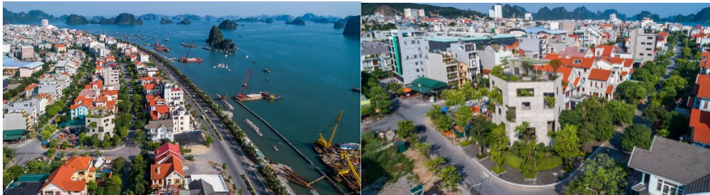
Figure 2.27: Hanoi Vietnam Source: (VTNArchitects, 2020)
