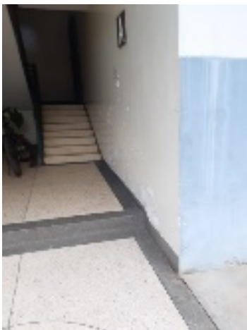
Figure 4.41: Bellway Court apartment staircase space Source: Author 2021
