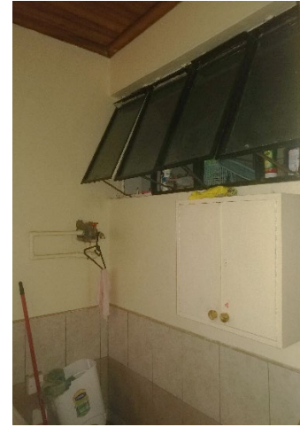
Figure 4.54: Ramis Court washroom ventilation occurring through the laundry Source: Author 2021
