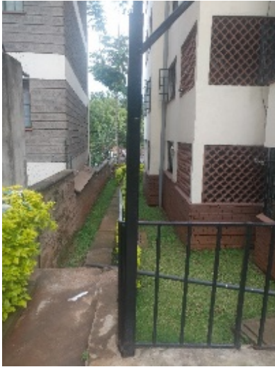
Figure 4.86: Sunning Hill apartment Brick screens Source: Author 2021
