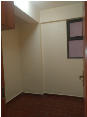
Figure 4.57: Kaisa Garden apartment finish Source: Author 2021
