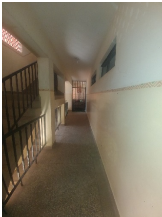
Figure 4.47: Ramis Court apartment staircase space Source: Author 2021
