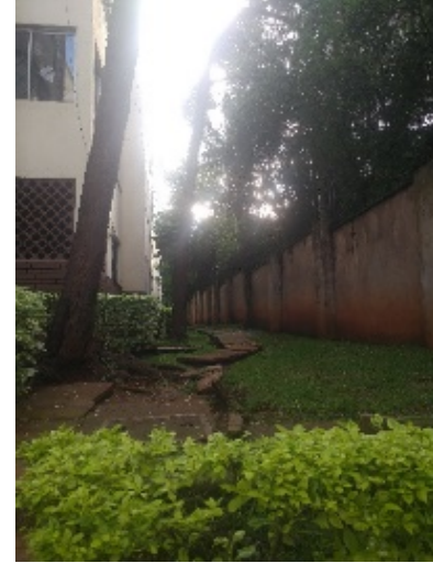
Figure 4.87: Sunning Hill apartment concrete pathway Source: Author 2021
