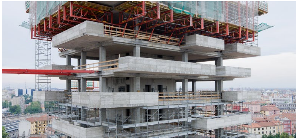
Figure 2.11: Bosco Verticale under construction Source: (Burrows, 2021)
