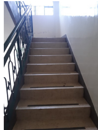
Figure 4.48: Bellway Court apartment staircase space Source: Author 2021
