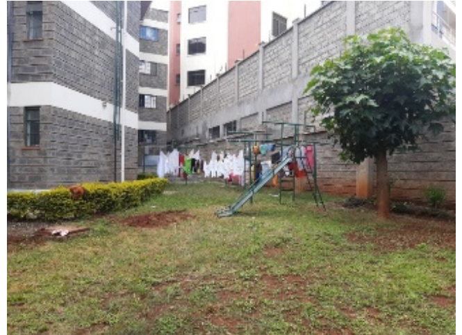
Figure 4.83: Bellway Court apartment masonry finish Source: Author 2021
