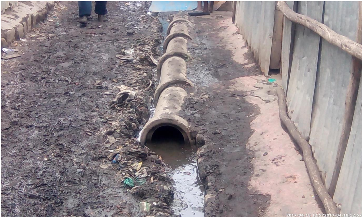
Figure 4-12: Culverts with thin width size in Mukuru kwa Ruben (Author, 18/04/2017)
