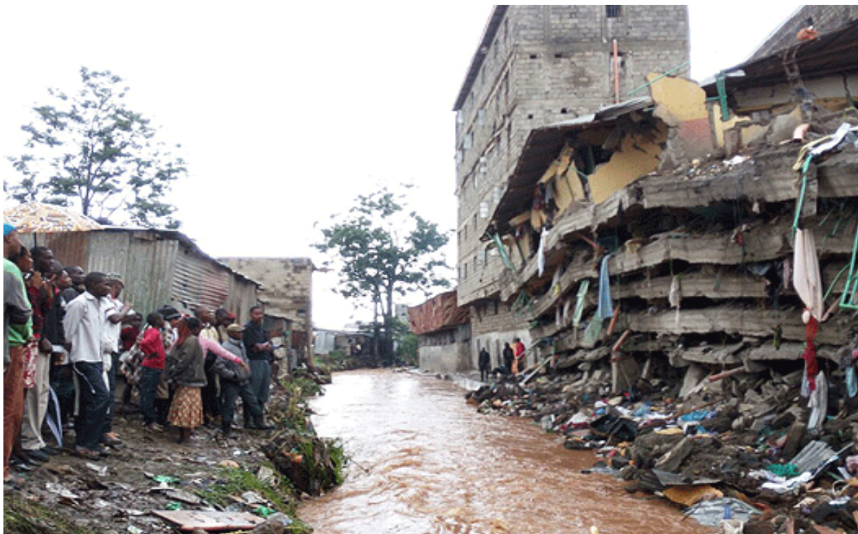
Figure 2: Collapsed building in Huruma in Nairobi, Kenya. (Source: Nation Media Group, 2016)
