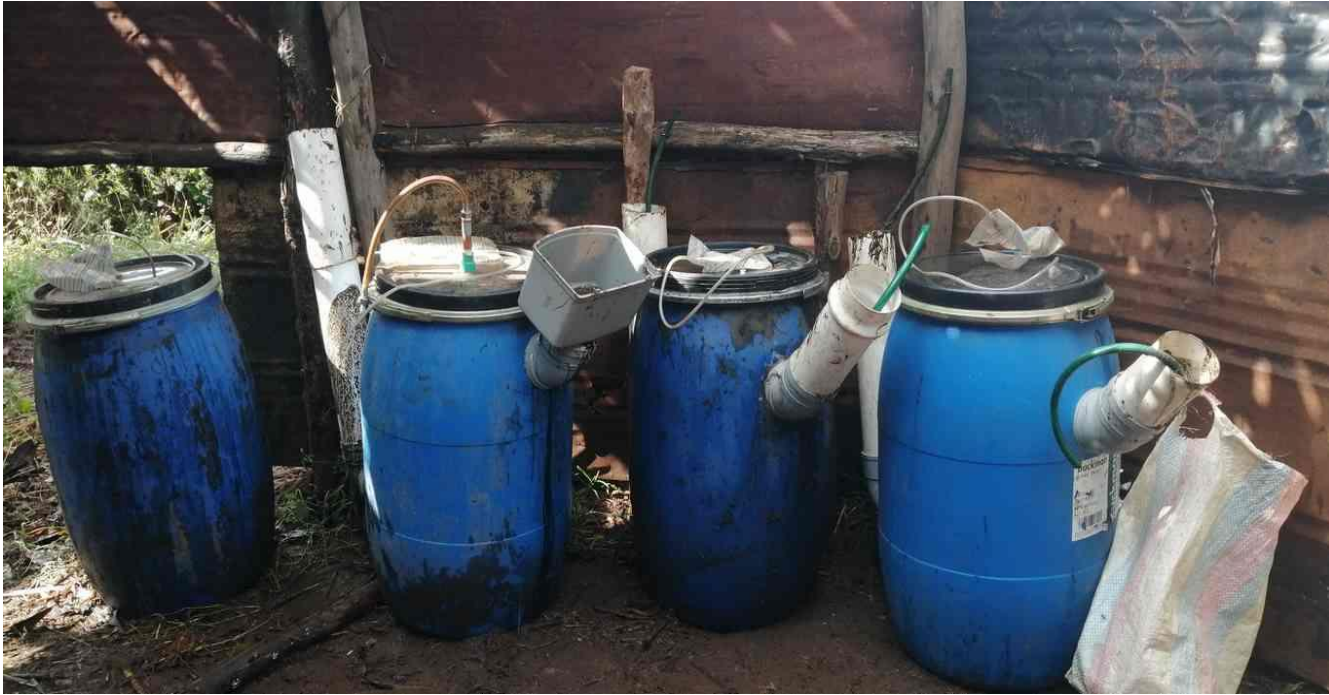
Figure 3.29: The biogas digesters
