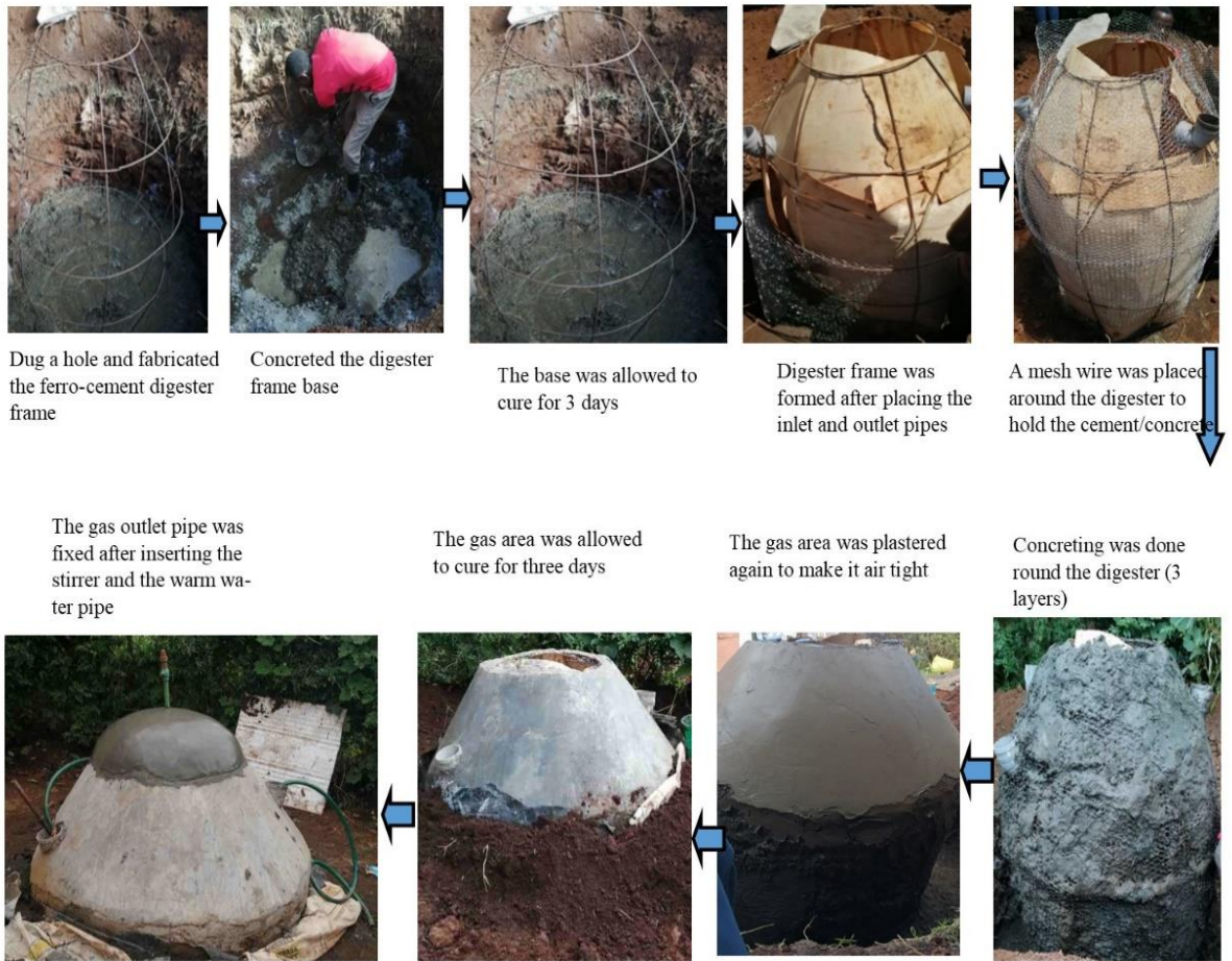
Figure 5.8: The steps followed in fabrication of Ferro-cement reactor
