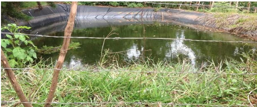
Plate 14: A Water Pan Constructed to Harvest Water.
