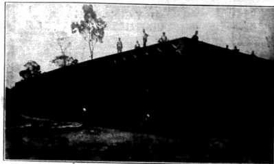
Nairobi's million gallon water storage tank. When the tank was partially filled for test purposes, the foundations, made of local stone, gave way.
