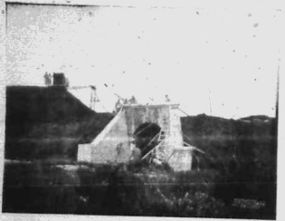
40 FT. CULVERT AND 25 FT. BANK AT MILE 29.
