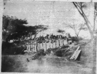
CONCRETE BRIDGE WORK FOR THE BIG KAJIADO.
