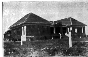
The new Club House.
