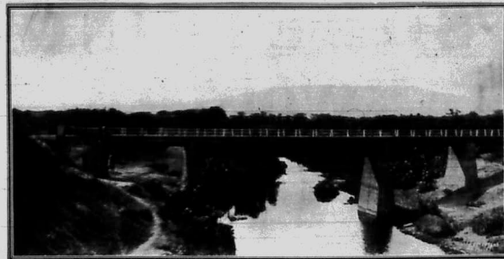
The new Masindi Bridge between Nairobi and Gilgil.
