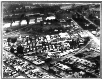
The sector of Nairobi between Duke Street and River Road seen from an aeroplane. Photographed by H. K. Hicks.
