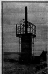
The machine used for marble production from marble chips.
