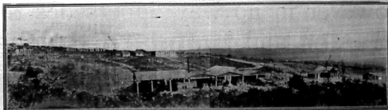
The site of the quarry and factory of the Kenya Marble Quarry Company near Kajjashi. A description of the work done appears elsewhere in this issue.
