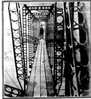
The gantry or viaduct, 300 feet long, in course of construction.
