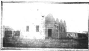
STANDARD BANK AT ELDORET, NEARING COMPLETION.
