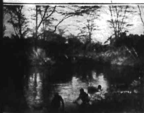
CLEARING A DAM, MAKINDU RIVER.
