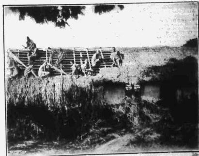
KIKUYU WORKMEN BUILDING A SWAHILI HOUSE Father Bantz, Cath. Miss., Mungu.
