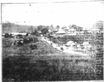
VIEW OF KILO FROM THE DOCTOR'S RESIDENCE SHOWING THE HYDRAULIC PIPE LINE RUNNING PARALLEL WITH THE ROAD HEADQUARTERS OF THE KILO MINING DISTRICT
