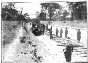
LAYING THE RAILS.
