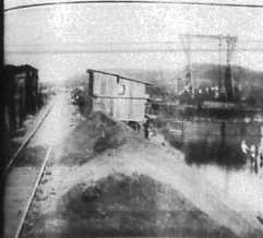
CONSTRUCTION OF BRIDGE AT MILE 50, MALAGABASSI.
