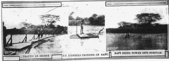
TRAFFIC ON BRIDGE
