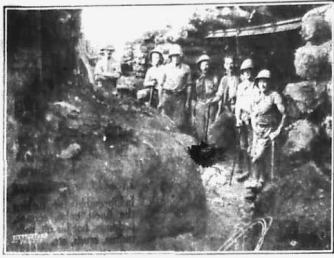
A TRENCH IN EAST AFRICA.
