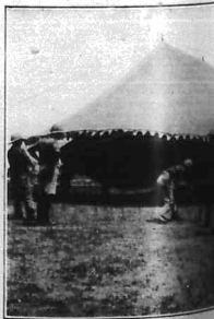
ERECTING A LARGE MAGAZINE AT M'BUYOL.
