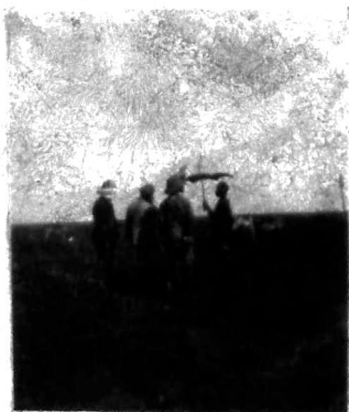
Finding position of Farm Boundary beacon with plane-table.
