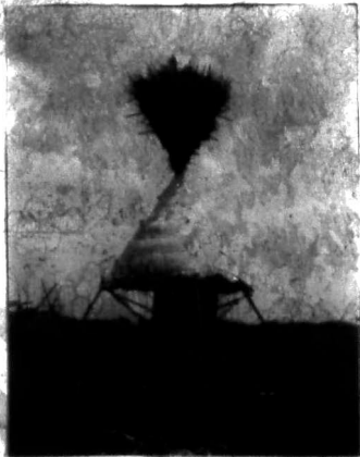
A wooden survey quadruped in a clearing of the bamboos on a ridge of the Mau Escarpment. The theodolite is centred underneath with a wind screen on the windward side.
