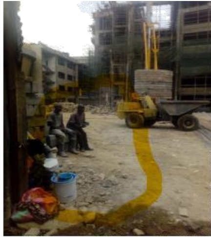
Fig.4.3 Poor Site Working Environment
