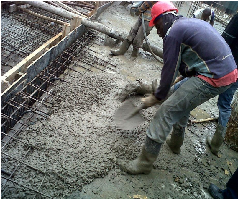
Image of concrete and reinforcement steel.
