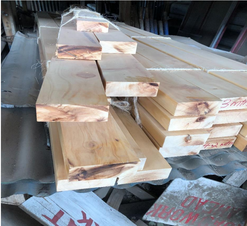
Timber for roofing trusses.
