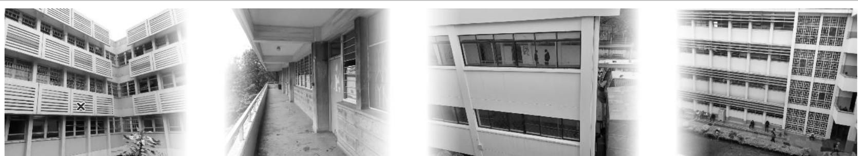
Figure 3-1: A photography illustration of the selected area of study (From left Horizontal concrete vents on N Block, Eastern balcony on U block, non-shaded façade and combined Eggcrate and aluminium louvers on C block).
