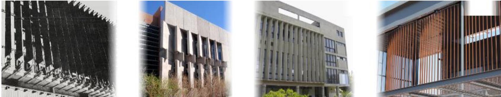
Figure 2-6: illustrations of vertical shading devices in use, Source: Arch daily 2020: Facades and solar control, Brise Soleil Systems for residential, commercial, corporate, hospitality
