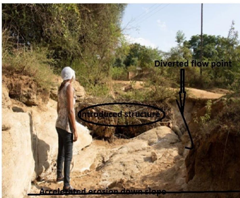
Figure 5.27: Accelerated downslope gully erosion
