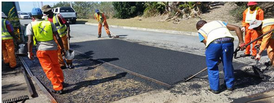
Plate 2-3: Section of the Northern Corridor under Maintenance
