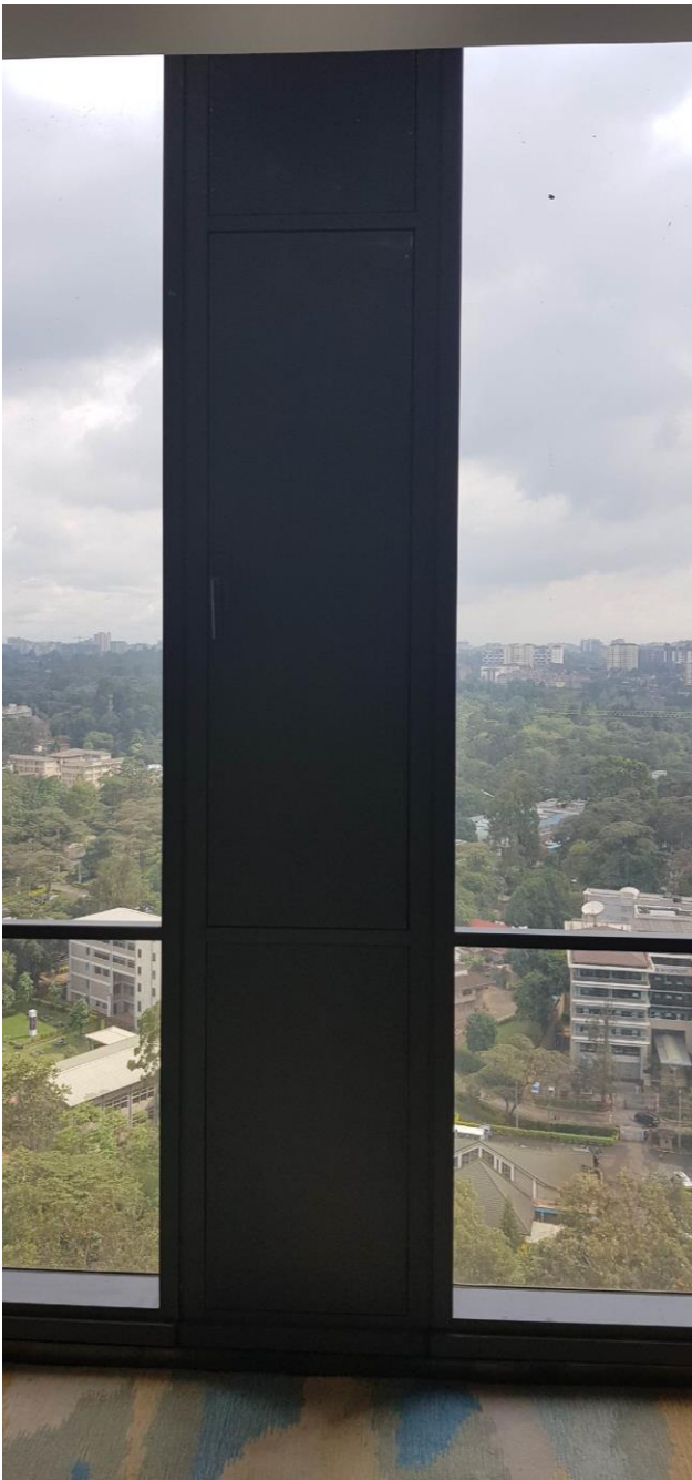
Figure 6.5: Operable pane at the Global Trade Centre Office Tower Source: Author
