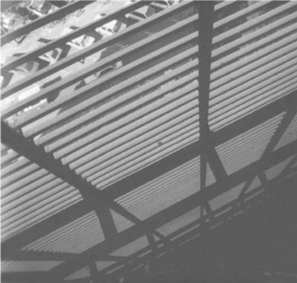
Figure 2.70: Interior view of the fixed louvres on the east façade of the atrium
