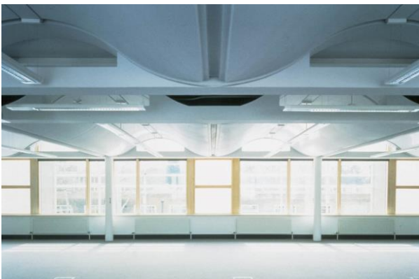
Figure 2.41: Perspective of sinusoidal roof used for cooling and heating Source: https://www.new-learn.info/packages/euleb/en/p6/index.html
