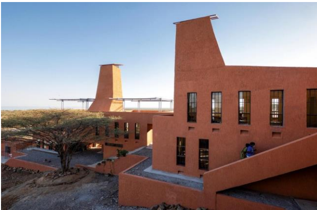
Figure 1.11: Thermal chimneys at the Startup Lions Campus in Kenya Source: https://www.archdaily.com/964238/startup-lions-campus-kere-architecture
