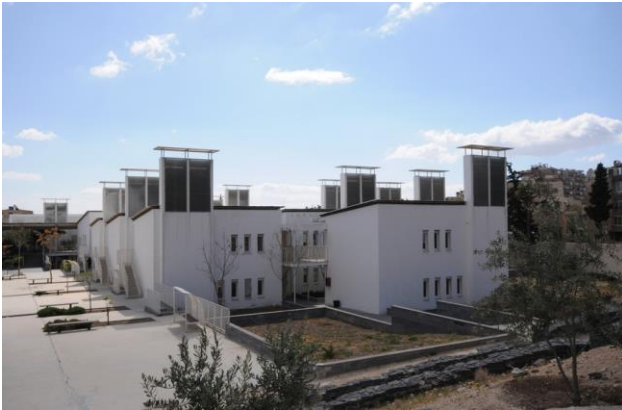
Figure 1.18: Thermal chimneys at Lycee Francais Charles de Gaulle in Damascus
