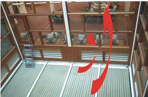
Figure 2.48: Ventilation grilles at Frederick Lanchester library Source: https://www.researchgate.net/figure/a-The-Frederick-Lanchester-Library-Coventry-University-Coventry
