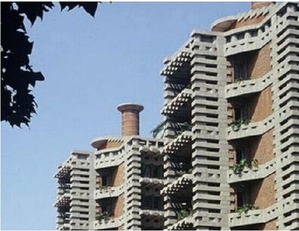
Figure 2.64: Perspective of sun shading elements at Eastgate Centre Source: https://www.researchgate.net/figure/Eastgate-Center-Harare
