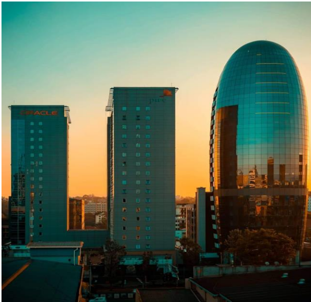
Figure 4.2: Perspective of Delta Corner Towers and One Africa Place Source: Author's archive
