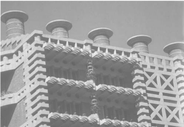
Figure 2.65: Perspective of sun shading elements at Eastgate Centre Source: https://www.researchgate.net/figure/Eastgate-Center-Harare
