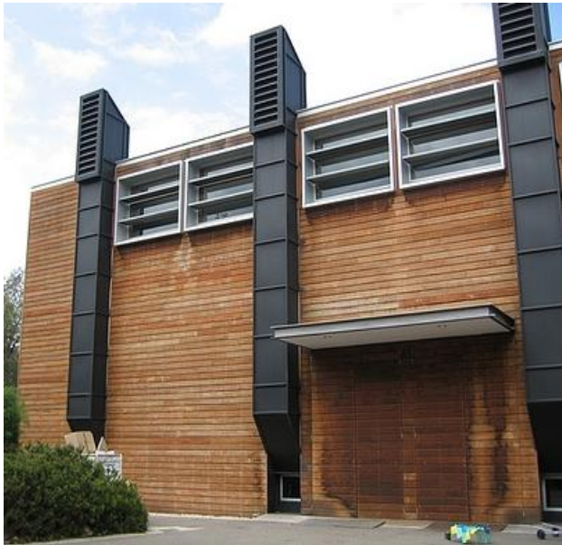
Figure 2.1: Thermal chimneys at Monash Science Centre in Australia Source: http://www.solaripedia.com/13/139/1263/monash_science_centre_wall.html
