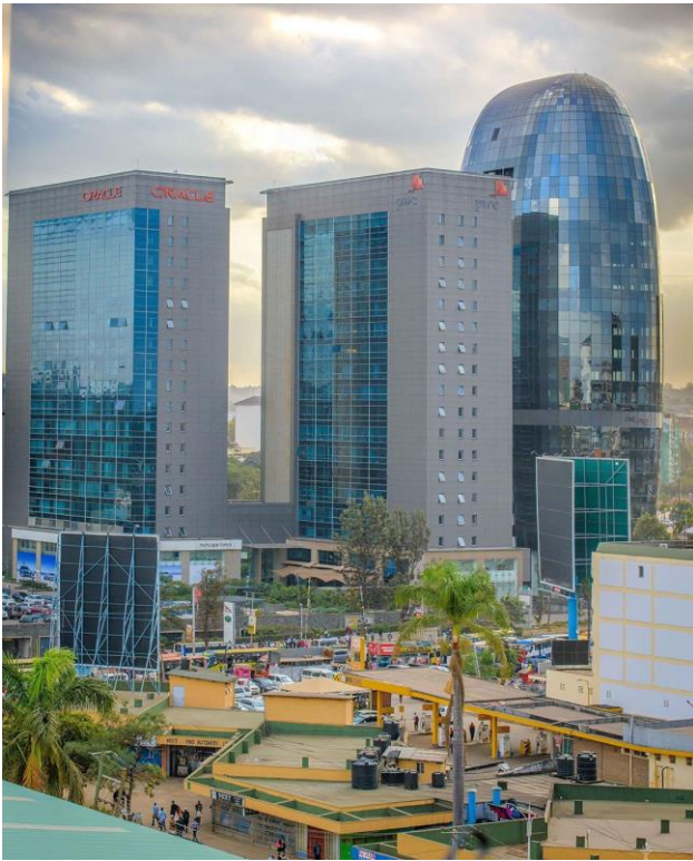
Figure 4.30: Perspective of Delta Corner Towers and One Africa Place Source: Author's archive
