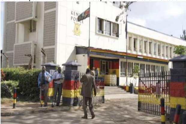
Figure 2.17: Perspective of a police station Source: https://www.kenyans.co.ke/news/50501-report-reveals-nairobis-7-most-dangerous-police-stations
