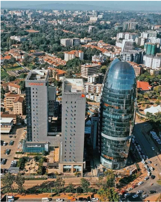
Figure 4.3: Perspective of Delta Corner Towers and One Africa Place Source: Author's archive
