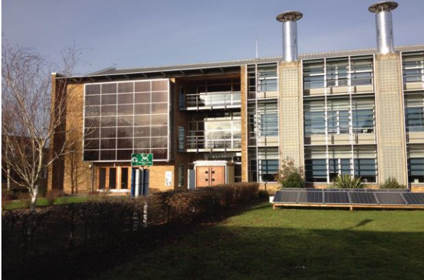
Figure 2.43: Perspective of photovoltaic system at BRE office Source: https://www.new-learn.info/packages/euleb/en/p6/index.html
