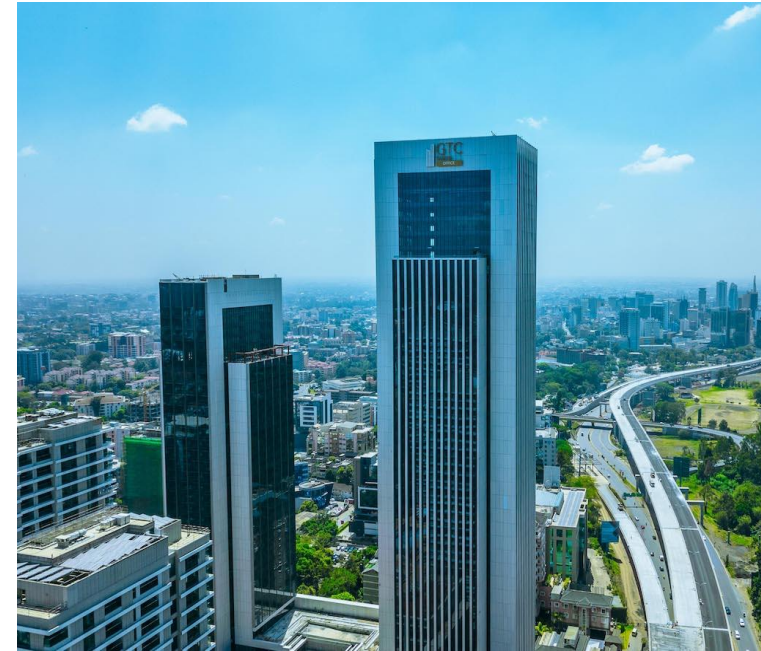
Figure 5.2: Case study 1- Global Trade Centre Office tower Source: Author's archives
