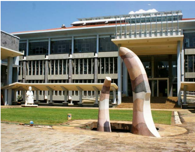
Figure 1.15: Auditorium at the Learning Resource Centre in Kenya Source: http://builddesign.co.ke/the-lrc/
