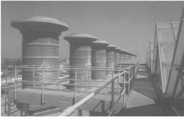
Figure 2.77: Perspective of thermal chimneys Source: https://www.researchgate.net/figure/Eastgate-Center-Harare
