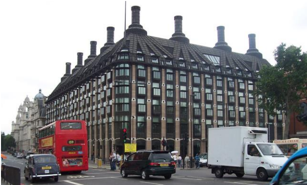
Figure 1.20: Thermal chimneys at Portcullis House in Westminster
