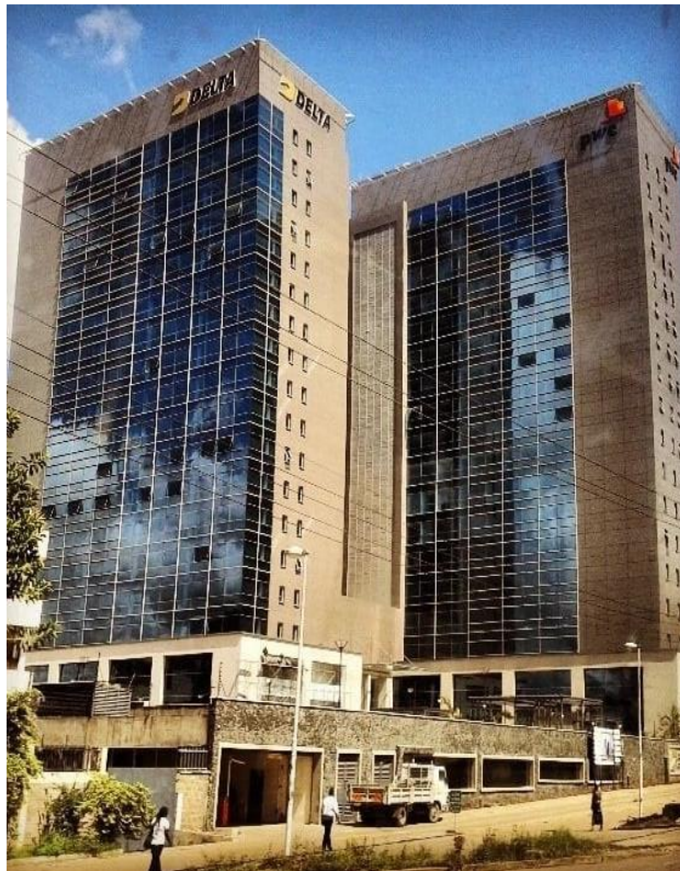
Figure 3.26: Perspective of Delta Corner Towers Source: https://baa-architects.com/office-corporate-projects/one-africa-place-nairobi-kenya/
