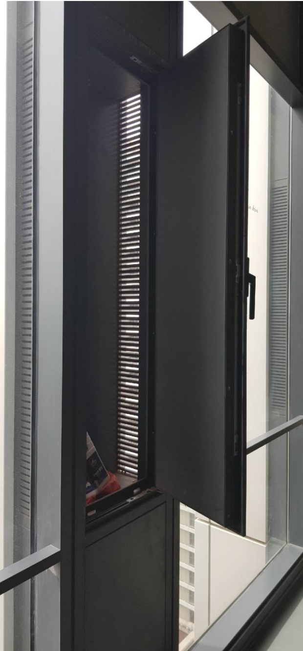
Figure 6.7: Operable pane and fixed louvres at the Global Trade Centre Office Tower Source: Author
