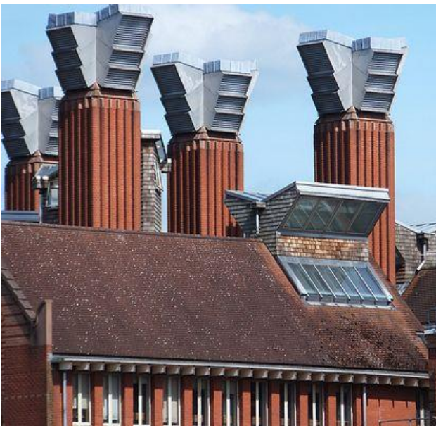
Figure 2.99: Perspective of roof mounted thermal chimneys at Queen's Building in Leicester Source: https://www.cam.ac.uk/research/news/back-to-the-future-of-skyscraper-design
