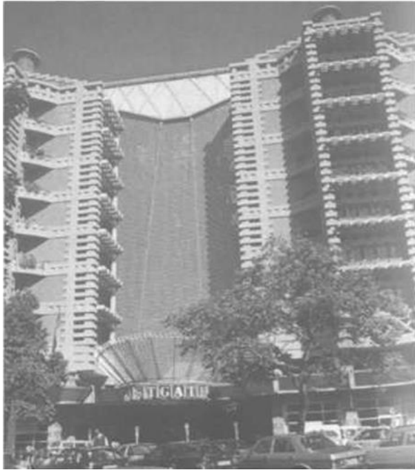
Figure 2.69: Exterior view of the fixed louvres on the east façade of the atrium
