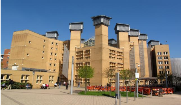
Figure 1.19: Thermal chimneys at Lanchester Library in Coventry
