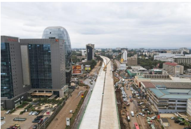
Figure 4.10: Perspective of One Africa Place and Delta Corner Towers Source: Author's archive
