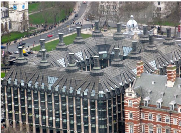
Figure 2.97: Perspective of roof mounted thermal chimneys at Portcullis House in Westminster Source: https://br.pinterest.com/pin/559642691174721243/
