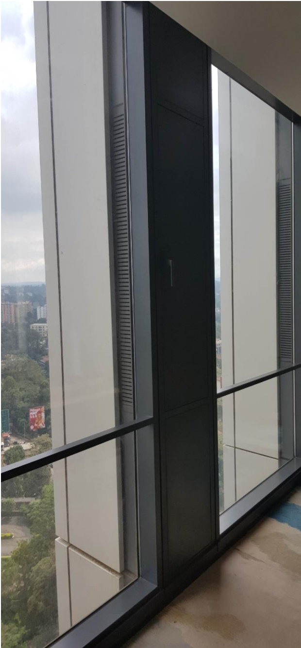
Figure 6.6: Operable pane at the Global Trade Centre Office Tower Source: Author
