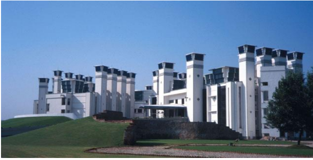
Figure 1.21: Thermal chimneys at Torrent Research Centre in Ahmedabad Source: https://www.archidev.org/spip.php?article1115&lang=fr
