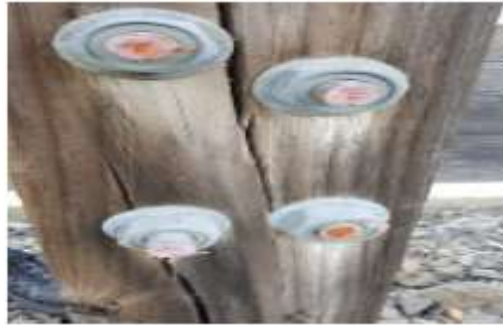
Figure 2.8: White Rust (Albanycountyfasteners.com, 2021).
