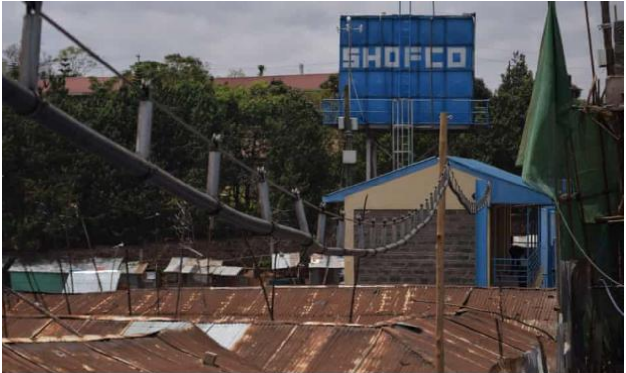
Plate 2.3 Aerial water piping system in Kibera
