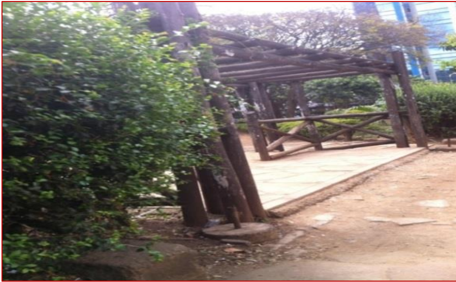
Figure 2.12: image of the new developed gate Source: Author, 2018
