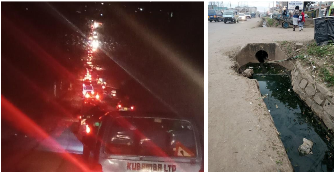
Figure 33: Magadi Road (left) traffic congestion and (right) poor drainage along the road
