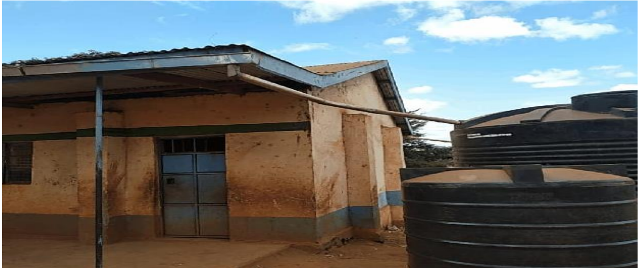
Figure 1: A section Kivai Primary school, Kaiti Constituency, Makueni County
