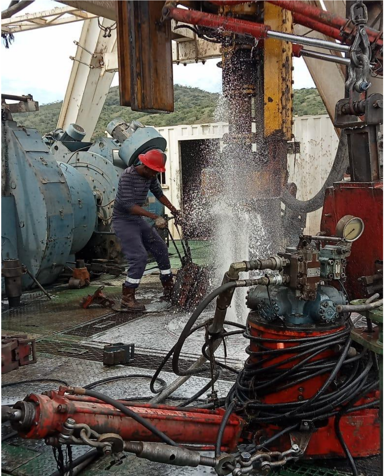
Plate 4. 3: Exposure to Hot Drilling Fluid and Sharp Edges from Drilling Machines
