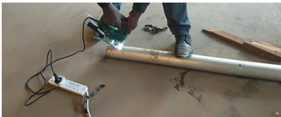
Figure 3.9: Sediment core retrieval
