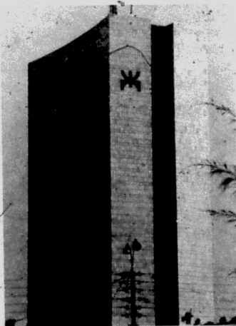
The 35-story Hotel Deux Février in Lomé is said to be losing $1 million per month
