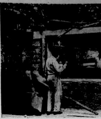
Workers size up the job after an explosion had ripped a showcase from the outside wall of the Chinese Embassy in Nairobi during Tuesday night. It was the second time the display had been destroyed.
