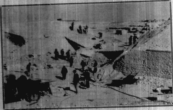
Repairing a bridge wrecked by the R.A.F. (Air Ministry Official Photograph)
